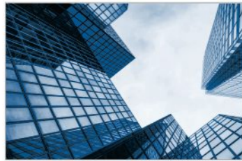
楼宇供水 Building water supply
